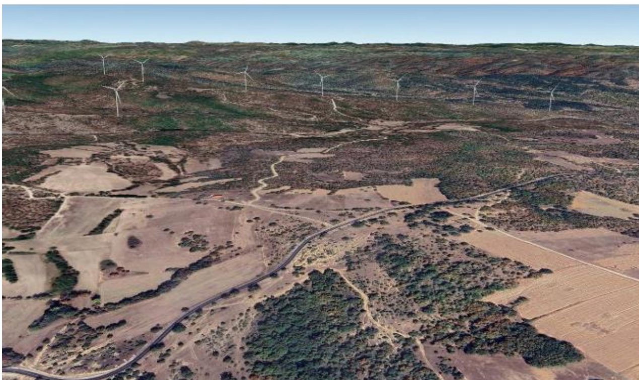
Picture 30: Panoramic view of the WPP with shooting direction north.
